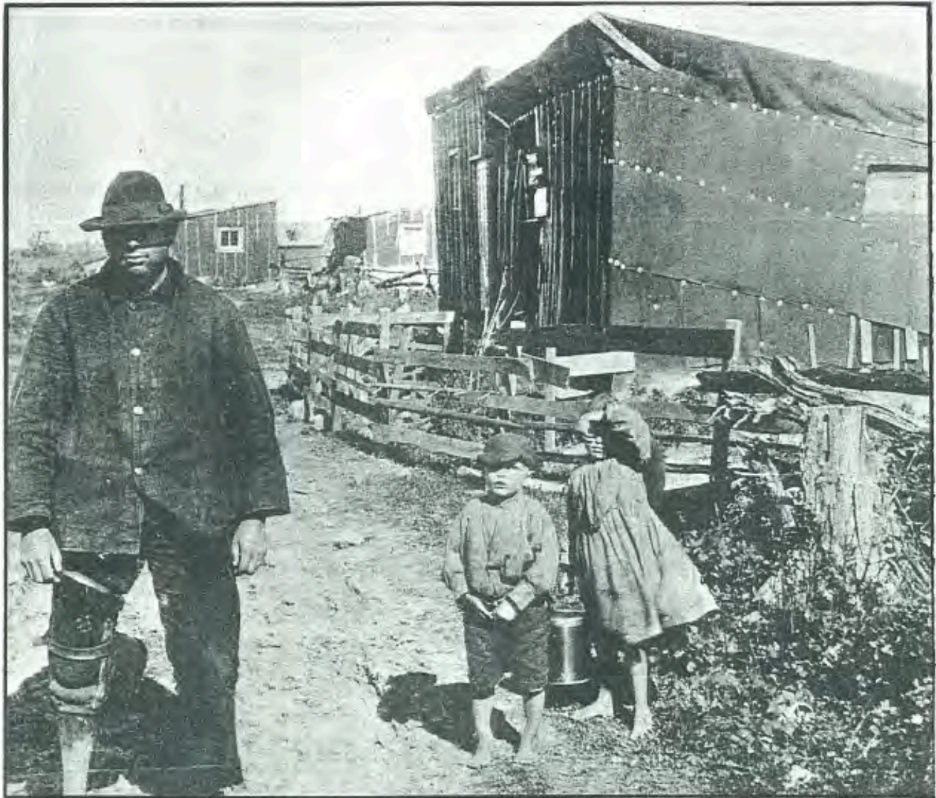
Typical iron mining town houses, Mesabi Range, Minn.
